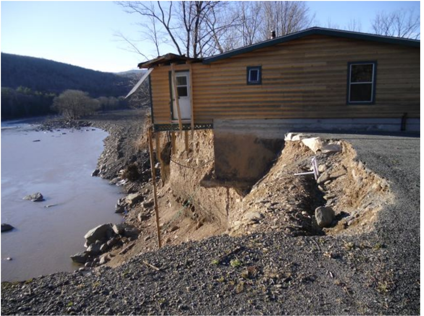
Upper Schoharie along Rt 23A with houses perched on glacial lake bed sediment
